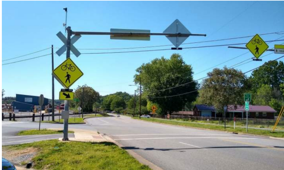
Trail Crossing Signs with RRFBs
